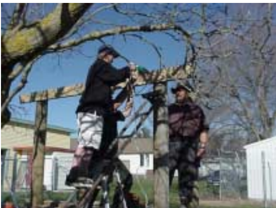
Drilling the roof supports
