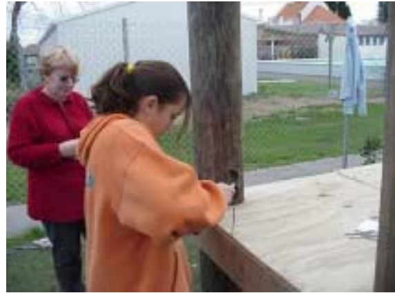
Nailing the floor
