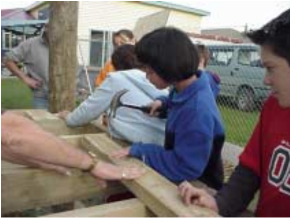
Pre-nailing the joists
