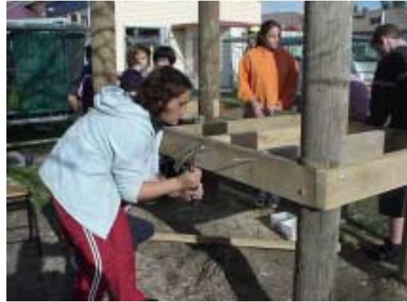
Hammering the floor joists
