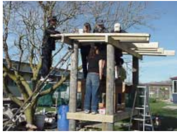
Placing the rafters
