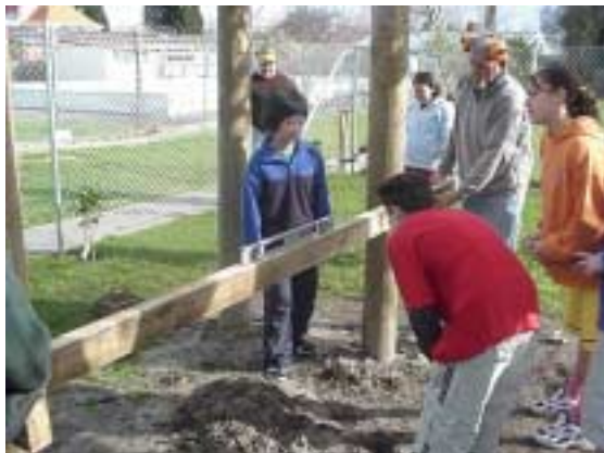
Checking the levels
